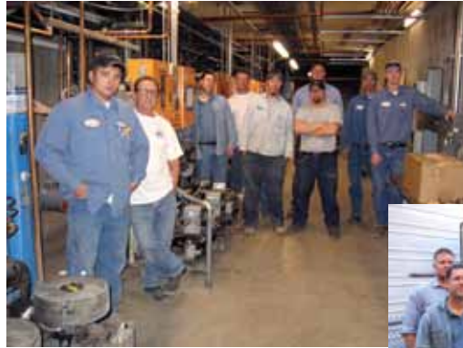
Fry's #19 equipment room
